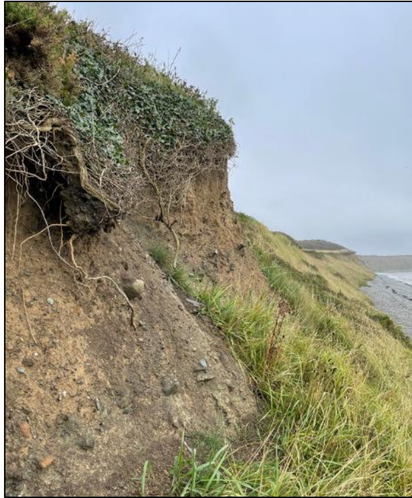
Plate 3: Back-scarp of landslide in cliff slope at landfall location.
