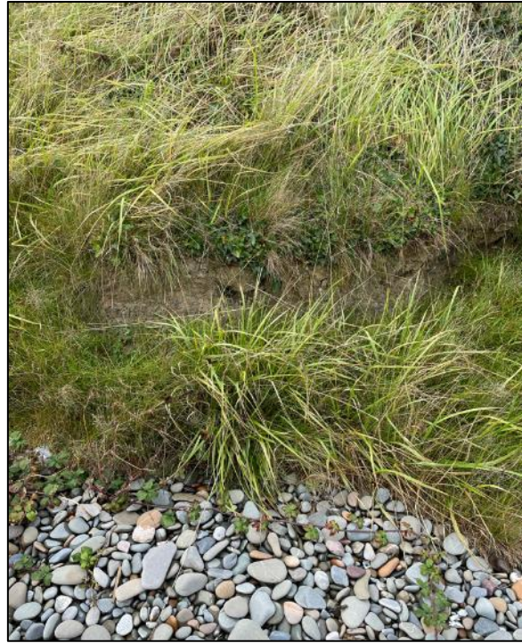
Plate 5: Minor erosion of toe of landslip material at landfall location.
