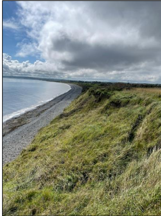
Plate 9: View south along crest of landslips in cliff slope.
