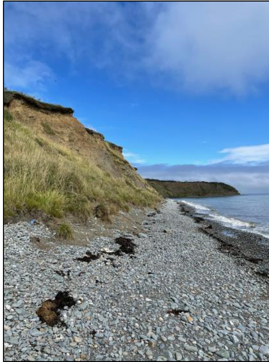
Plate 7: Increase in extent of active landslip in cliff slopes about 0.5 km north of landfall location.
